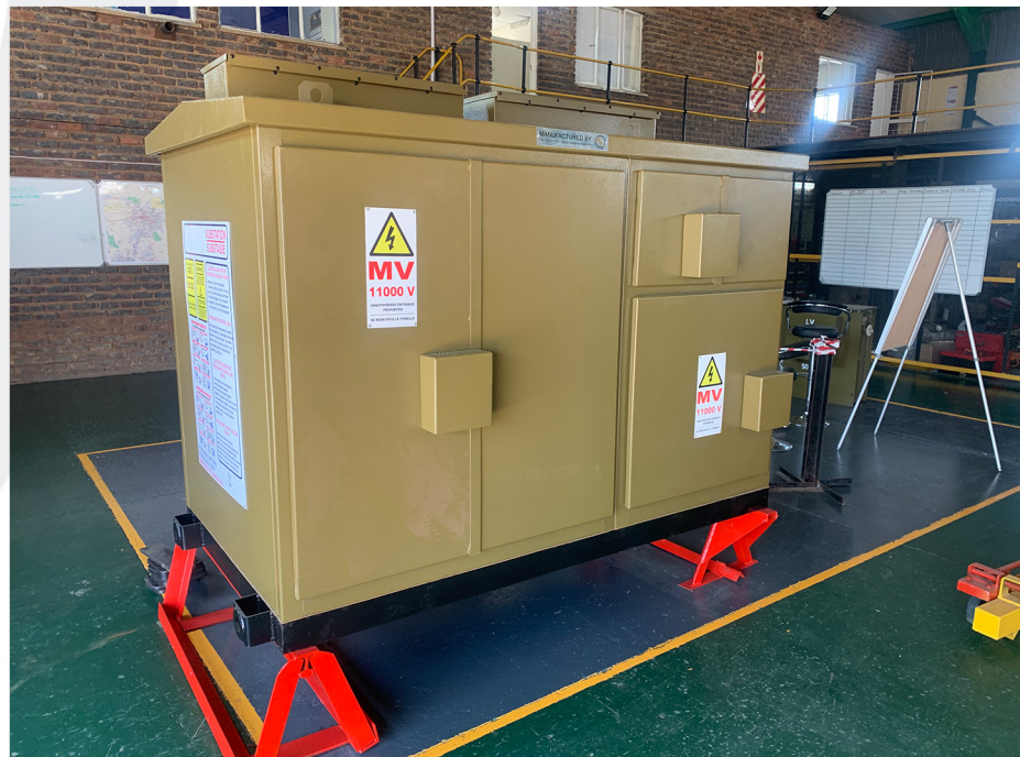
Bulk Metering Kiosk, Fitted with multi-function power quality analyser with wifi and cellular
