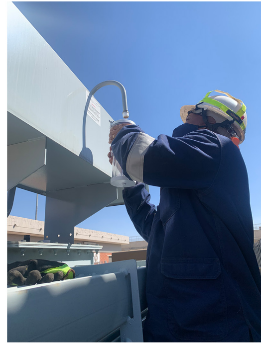
Site Service - Replacing Breather
